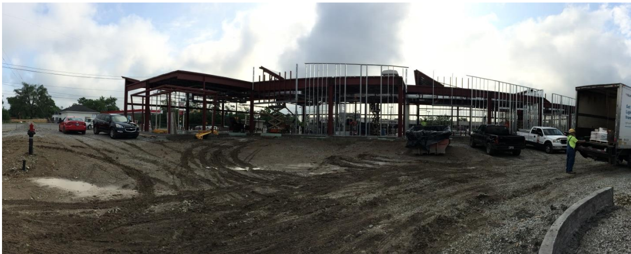
Project Site on July 30, 2019 Panoramic view of the west side of the building.
