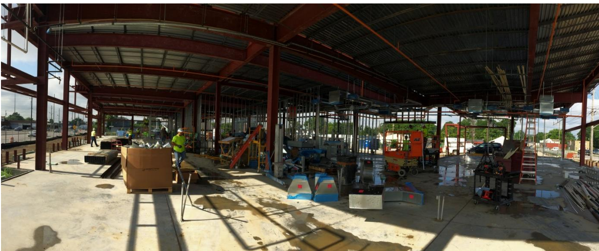
Project Site on July 30, 2019 Interior panoramic view from the east entrance at Sherman Drive.
