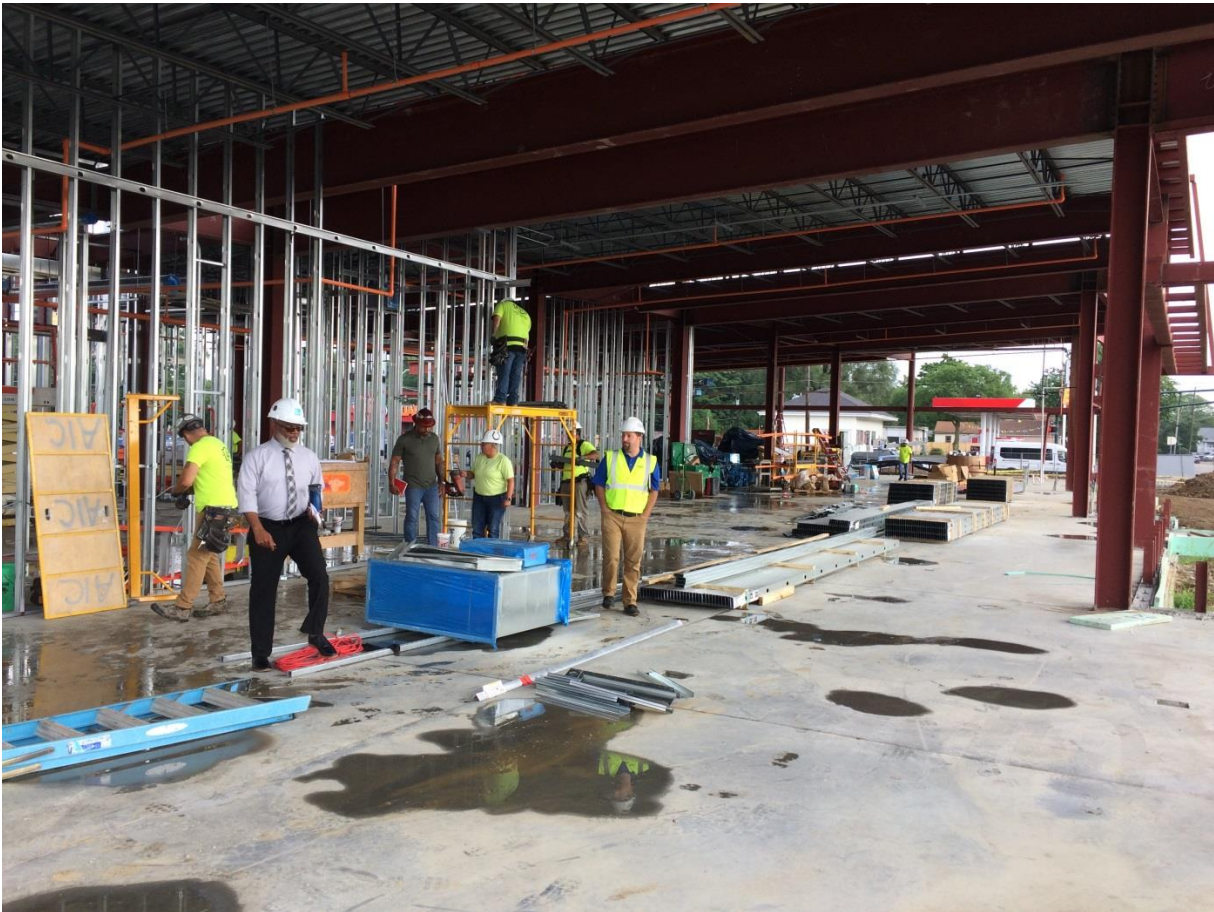
Project Site on July 30, 2019 Interior view of the Children's Area looking north.
