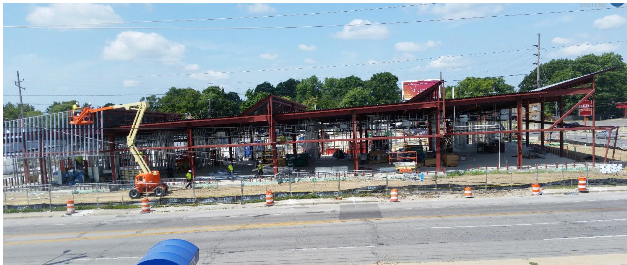
Project Site on August 8, 2019
