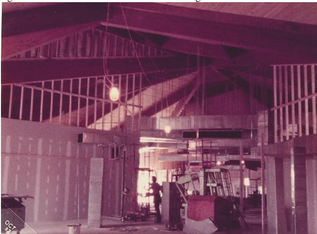
View of the Interior Laminated Wood Structure During Construction dated October 1982.
