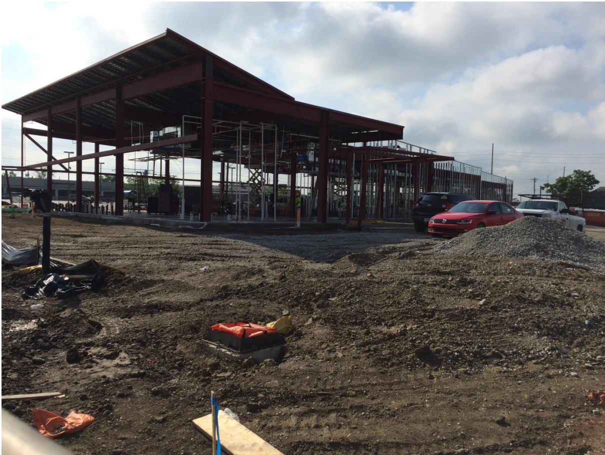
Project Site on July 30, 2019 View of the west entrance from 25 th Street.
